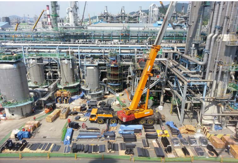
C2 splitter tray revamp installation
