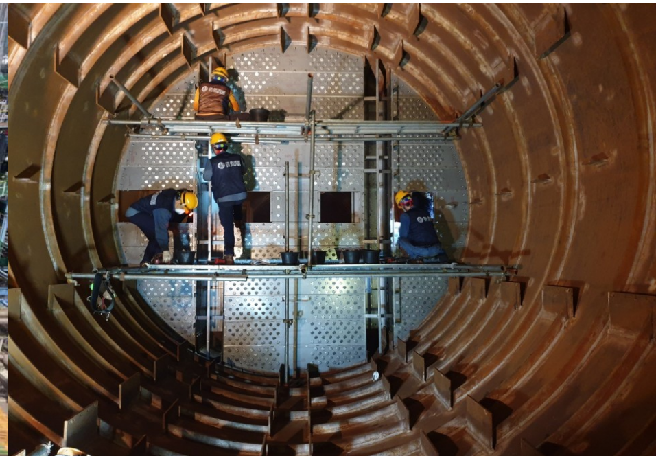
Horizontal tray installation
